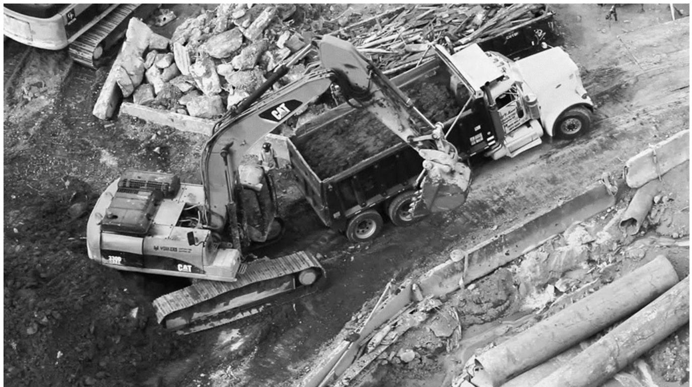
See this image and how deadly the end could be for this worker standing between those two heavy equipment in operation and one of them backing up. A backover incident occurs when a backing vehicle strikes a worker who is standing, walking, or kneeling behind the vehicle. These incidents can be prevented.
