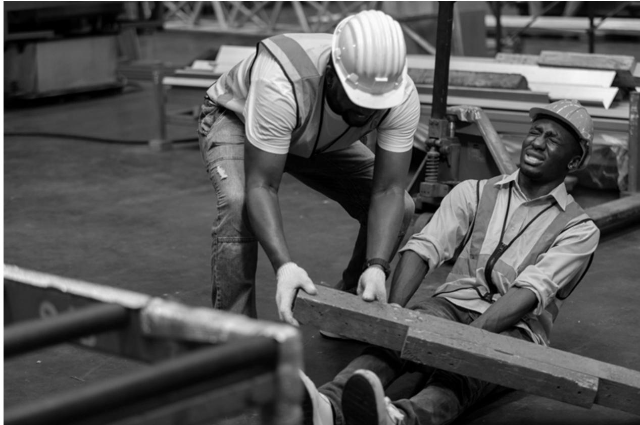
One worker appears to be injured after being struck by a heavy object, possibly a beam or board, and is sitting on the floor in pain. The object may have fallen or been mishandled, suggesting poor material handling practices or a lack of hazard awareness. No visible barriers, signage, or lifting equipment are in place, and the workspace is cluttered, increasing the risk of struck-by incidents.
