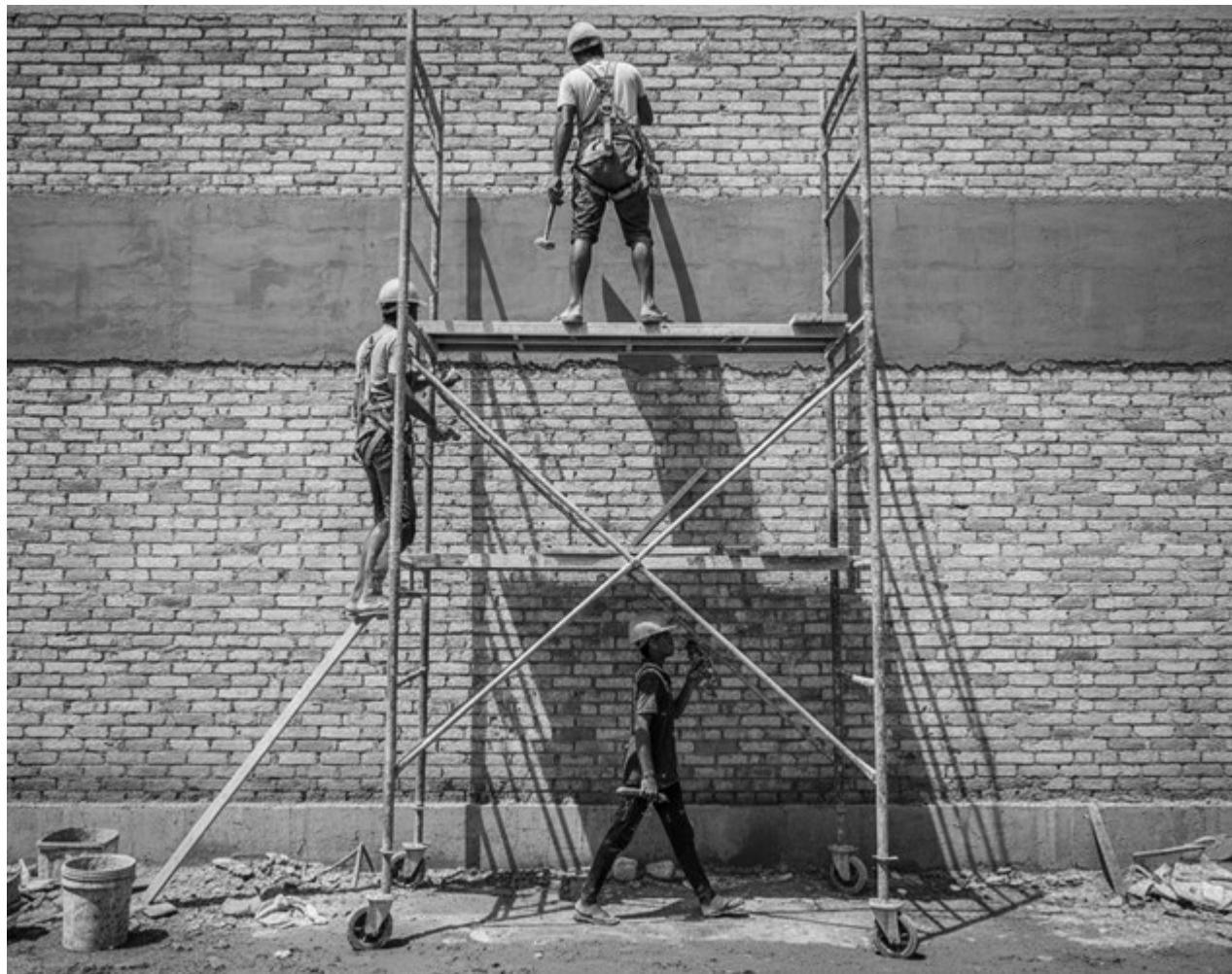
This image captures a highly unsafe scaffolding setup. The base appears unstable, supported by a makeshift wooden plank, and the wheels aren't locked. Workers are climbing the frame instead of using a ladder, and although they wear harnesses, there are no visible anchor points or fall arrest systems in use. One worker walks underneath the scaffold—a major struck-by hazard if tools or materials fall.
