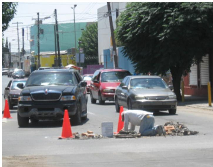
A couple of orange traffic cones are the only thing standing between this worker and the vehicles traveling at 45 mph in the intersection where this picture was taken. Not wearing a high-visibility vest adds insult to injury.
