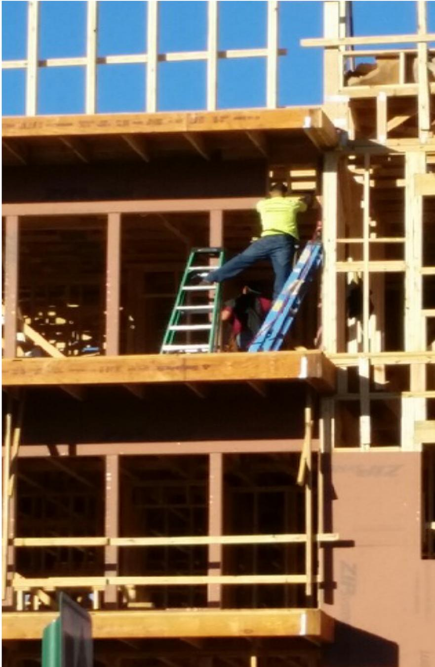
Doubling up on ladders is never a good thing. This construction worker was photographed standing with one foot on each of two stepladders at a Florida building site. If one of those ladders went sideways, this worker could fall backwards and end up permanently grounded. (Naval Safety Center)
