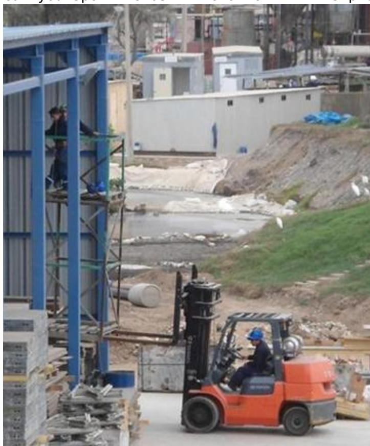
It's a bit hard to make out, but the workers in this picture are using the forks of the forklift to support one end of the scaffold another worker is working on. This is an unstable and dangerous arrangement that violates OSHA requirements for supporting scaffolds (Sec. 1910.28(a)(2) for General Industry, Sec. 1926.451(c)(2)(v) for Construction).
