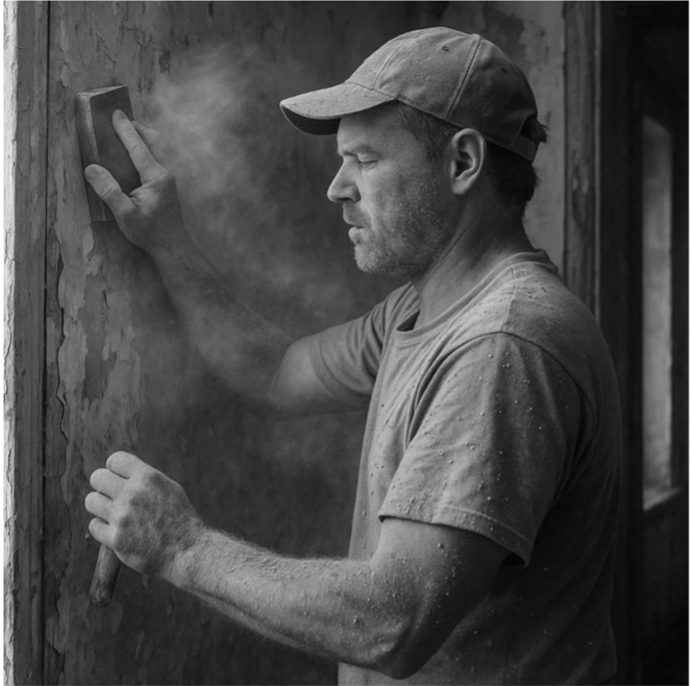
The worker is sanding or scraping painted surfaces without any respiratory protection, gloves, or protective clothing, generating a large amount of dust. If the paint contains lead, this creates a serious inhalation and ingestion hazard. Lead dust can enter the lungs or contaminate hands, clothing, and nearby surfaces—leading to chronic lead poisoning, which affects the nervous system, kidneys, and reproductive health.
