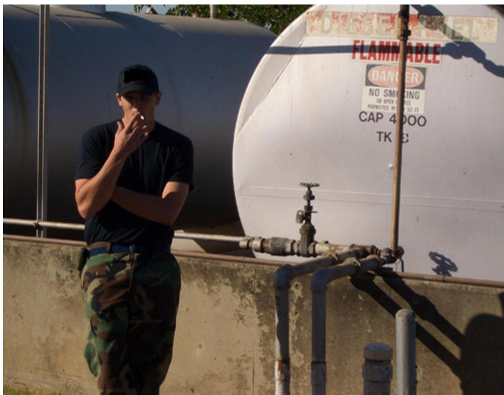
The good news is that the white fuel storage tank in the background is marked with the proper NO SMOKING warning. The bad news is that the worker has literally turned his back on the warning while puffing blissfully away.
