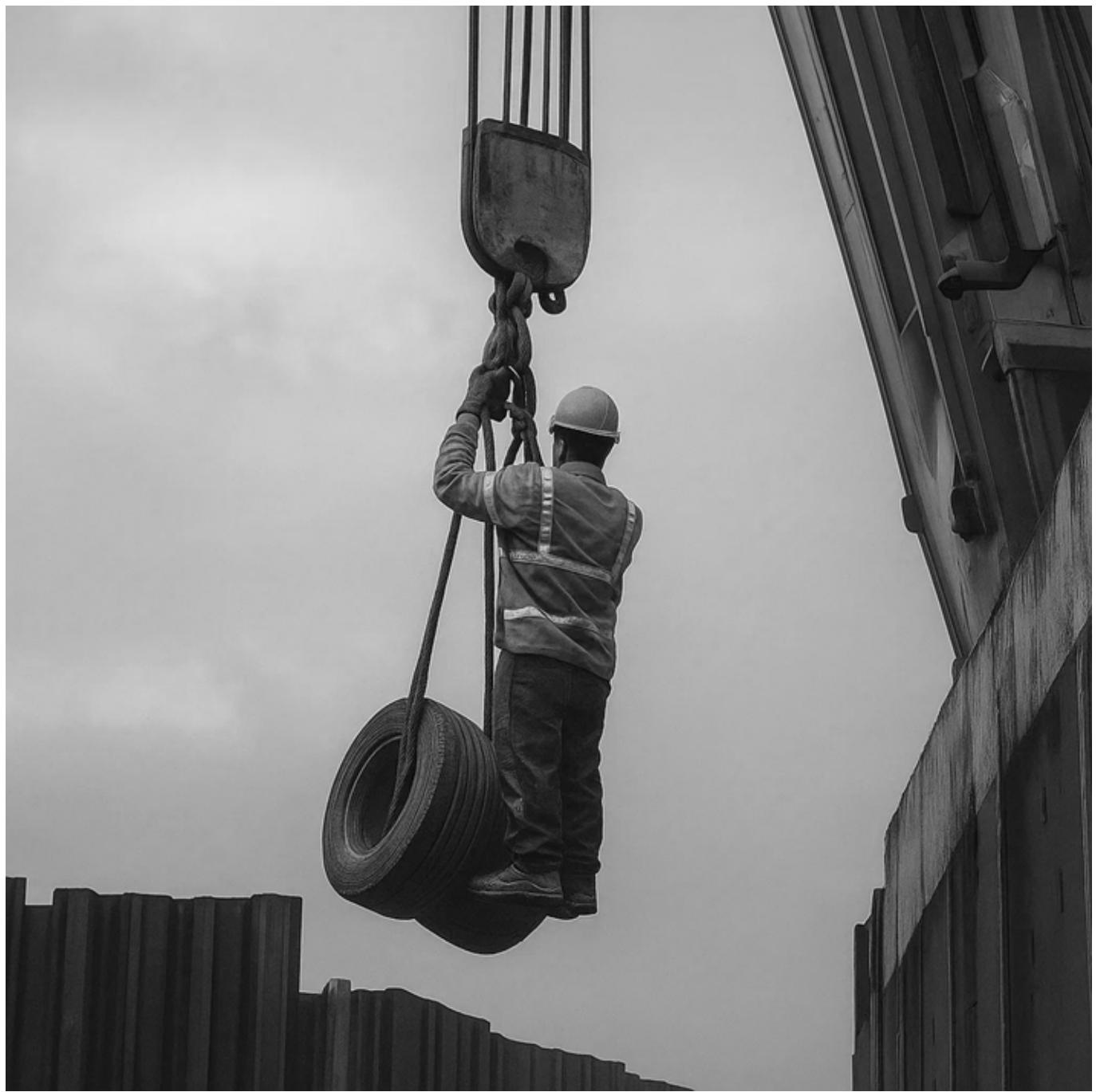
The worker is standing on a suspended load (a tire being lifted by a hoist), which is extremely dangerous. This behavior violates standard hoisting safety protocols. If the load shifts, swings, or fails, it could result in serious injury or death. Additionally, this action puts the worker at risk of a fall from height with no visible fall protection in place.
