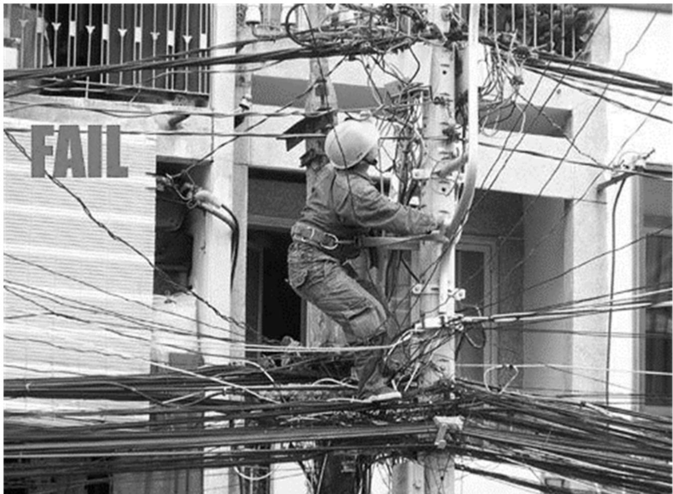
**What's wrong in this picture?** There is an electrician working in direct contact with exposed electrical power lines.
