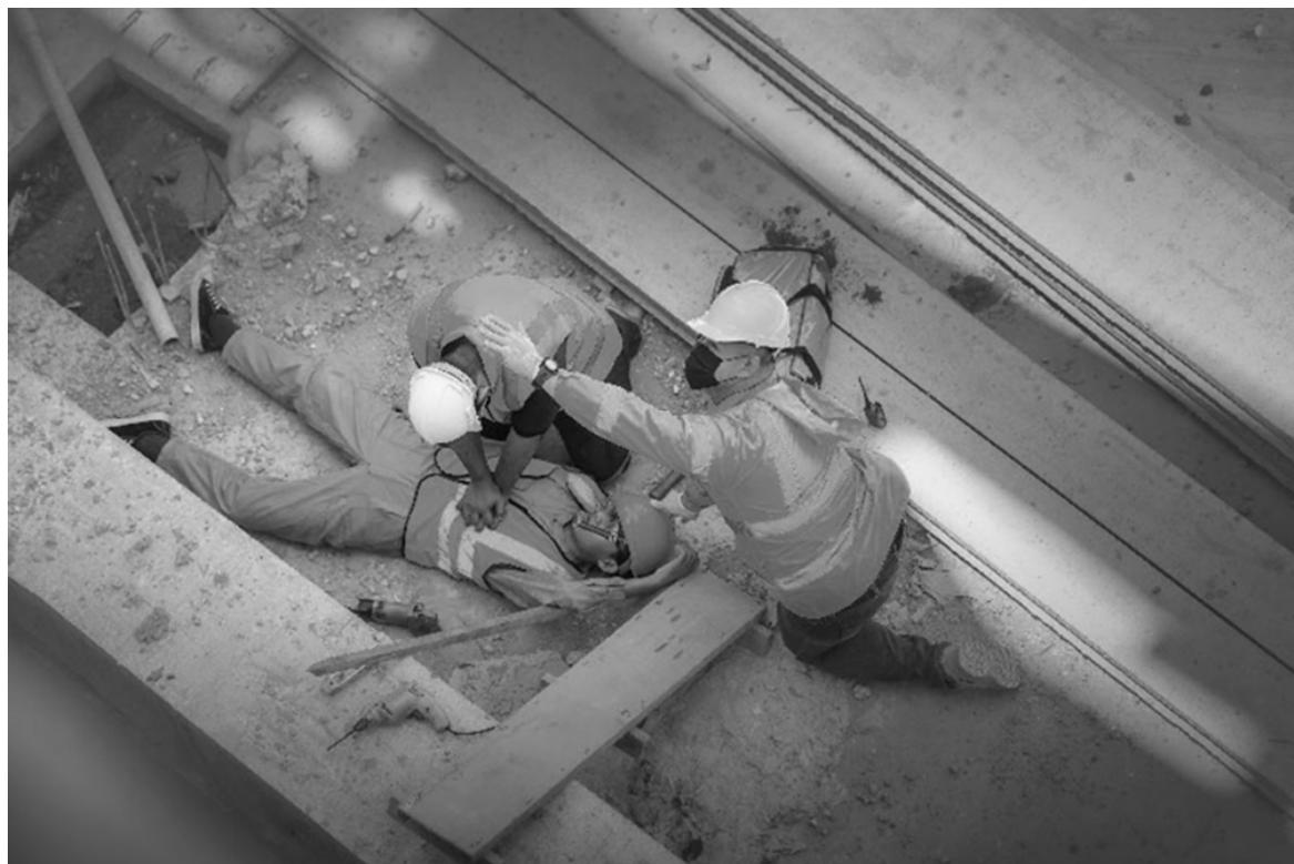
The worker is lying injured on a concrete surface, likely due to an electrical shock or fall related to unsafe tool use or exposed power sources. Tools are scattered on the ground and no barrier or warning signage is visible, indicating poor housekeeping and hazard control. There's no sign of ground fault circuit interrupters (GFCIs) or protective measures to prevent such incidents.
