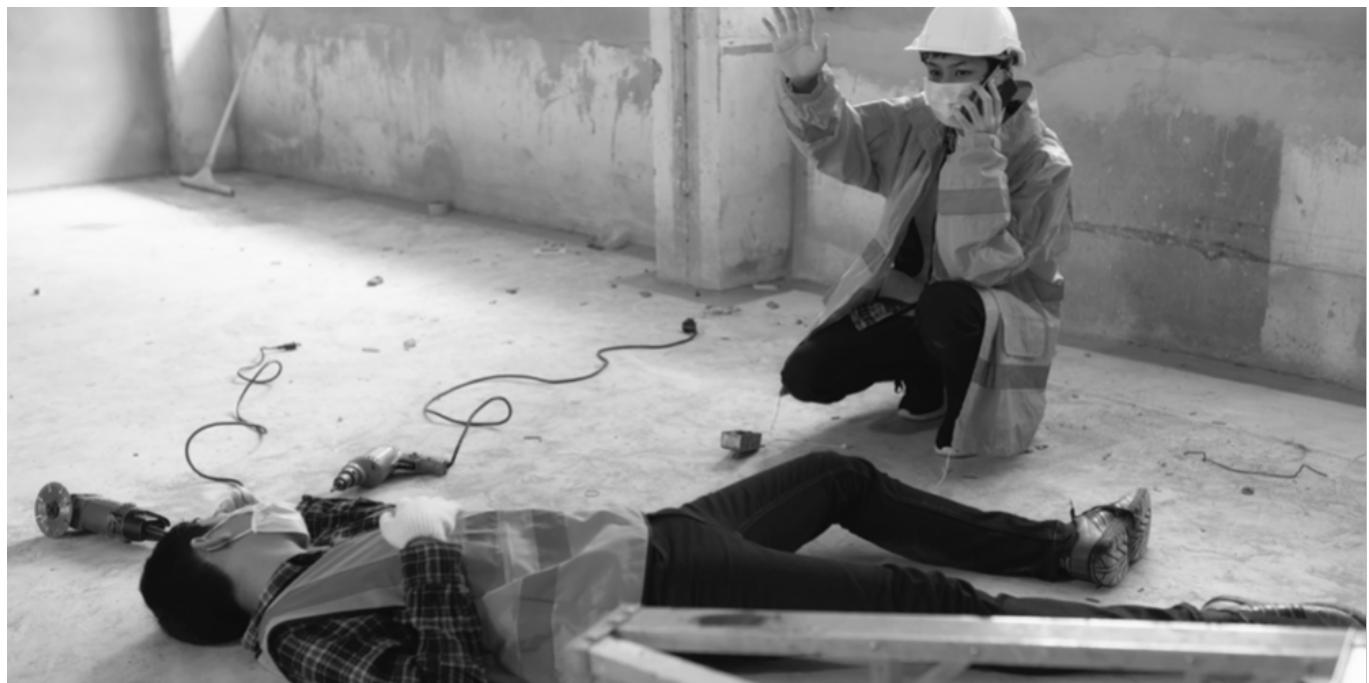
The worker is lying on the floor with power tools and exposed cords nearby, suggesting a possible electrical shock or trip incident. The tools are not secured or unplugged, and no lockout or warning measures appear to be in place. The surrounding work zone is cluttered and lacks visible hazard signs or physical barriers to prevent entry.
